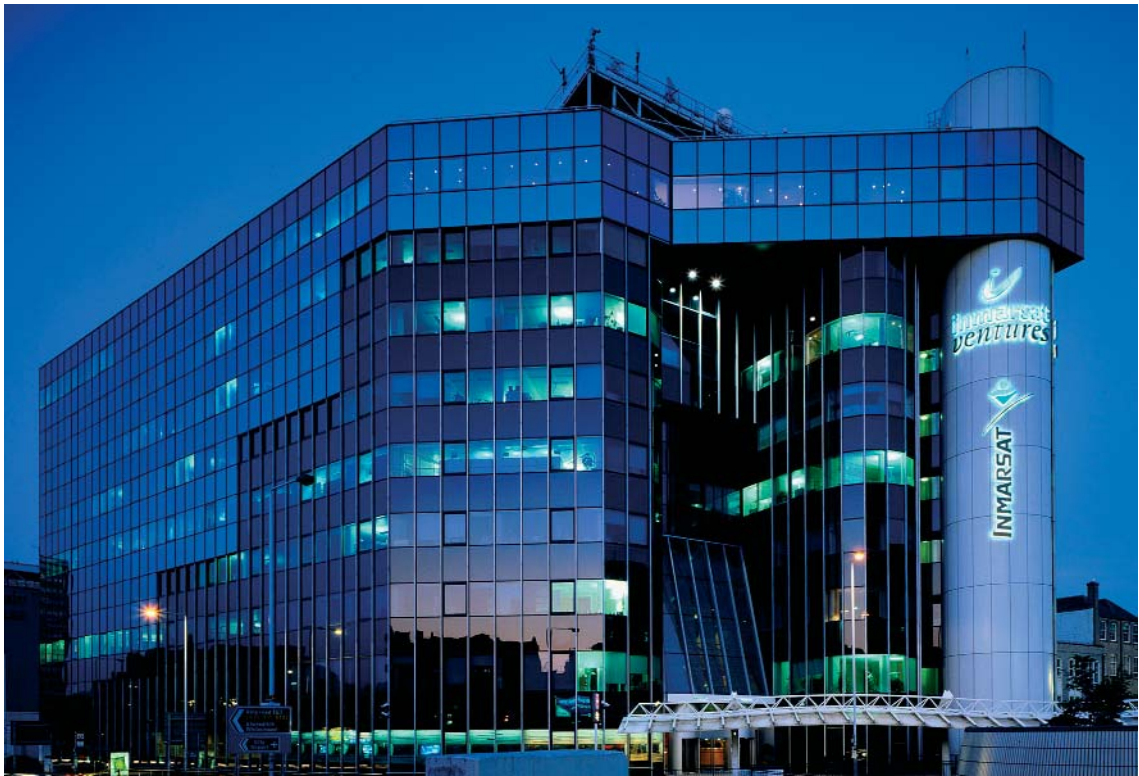
Figure 1 INMARSAT Headquarters in London. It accommodates the administration, as well as the operation centre
