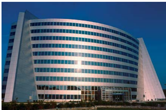
Figure 8 The headquarters of Telenor Satellite Services (TSS) US operation at Rockville, Maryland
