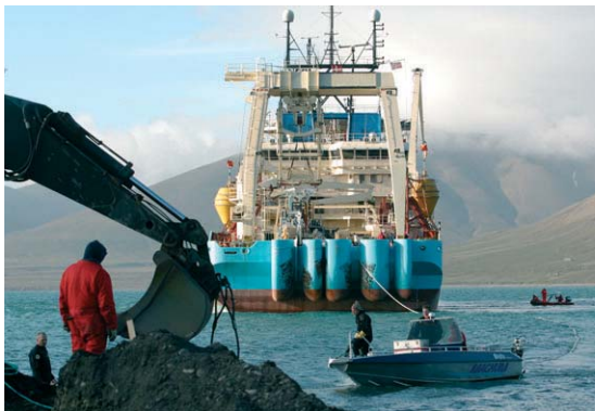
The final metres of the fibre are put in place by the cable ship on the sea floor reaching Spitzbergen in August 2003
