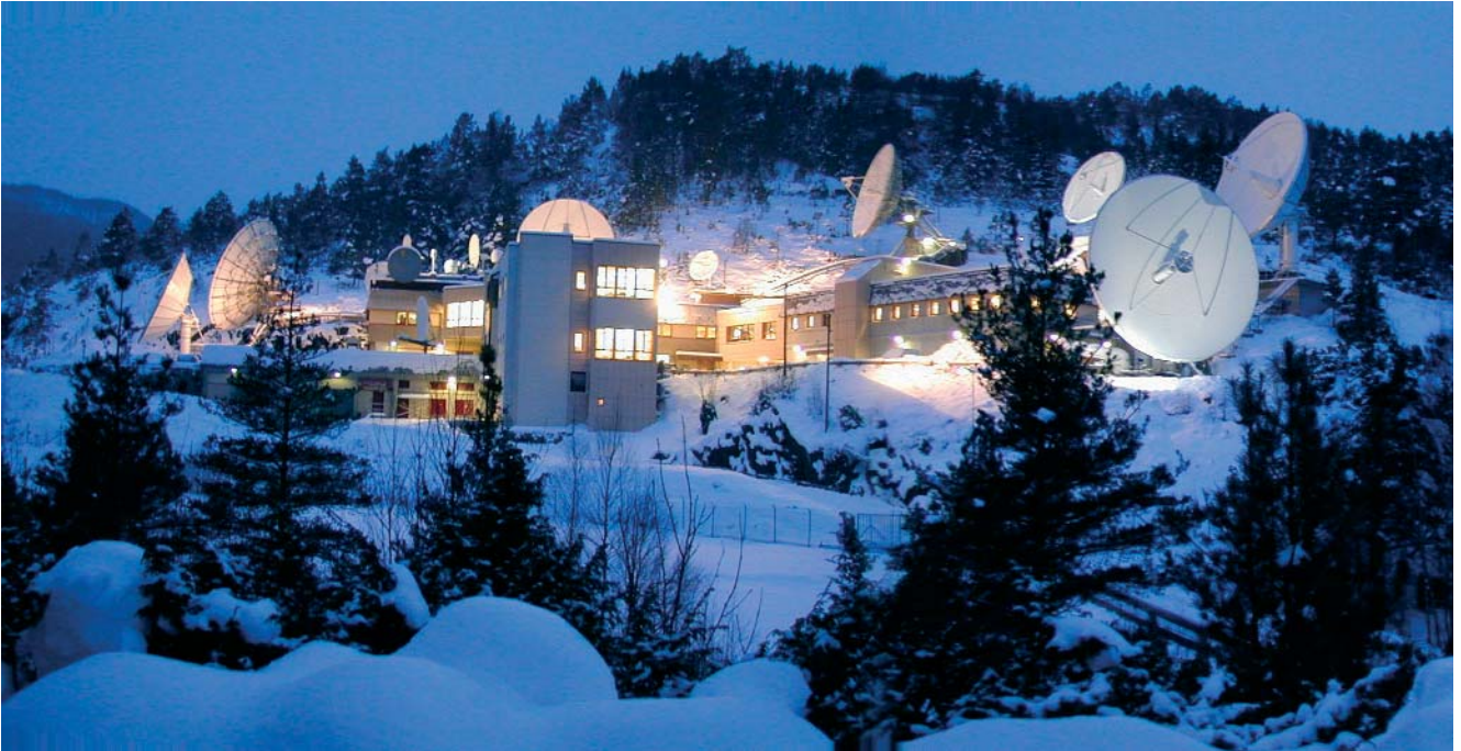
Figure 7 Eik earth station (Photo: Ole Gunnar Mosvold)
