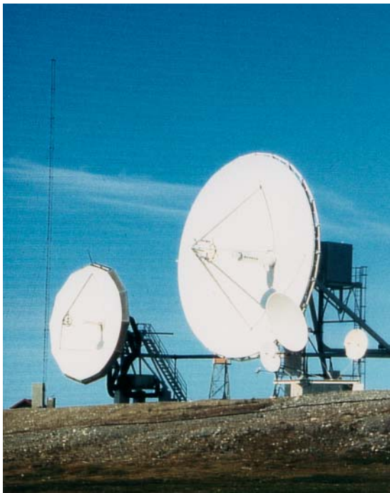
The satellite antennae at Isfjord radio has a diameter of 13 metres. Notice that the antennae is nearly pointing parallel with the terrain. This is because the elevation angle is only approximately 3 degrees
