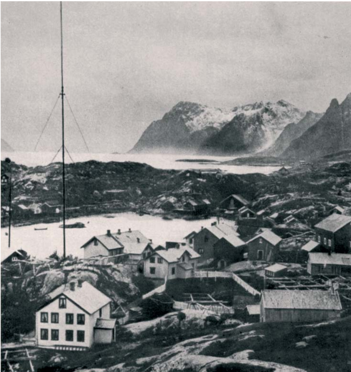
The picture shows Sørvågen Radio in 1906. Originally, both Sørvågen and Røst had 50 m radio-towers made of spliced spruce. It was secured by 28 wires in seven groups. The masts were approximately 40 m from the telegraph building. The upper part of the mast in Sørvågen was destroyed by storms several times, and the height was reduced to 40 m. (Photo from T. Rafto [4])
