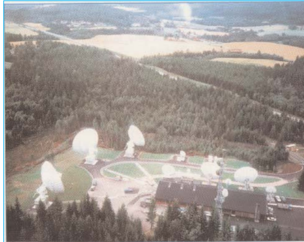
Figure 9 Nittedal earth station outside Oslo, Norway
