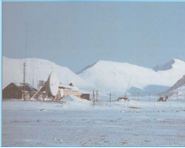
Figure 7 The earth station at Isfjord Radio, Spitzbergen, 78° North. At this station the maximum elevation angle towards a geostationary satellite is 3.1°
